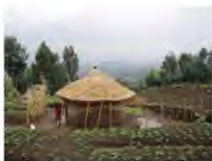
A typical rural dwelling of wattle and daub (a framework of woven sticks plastered with a mud/dung mix); those are potatoes growing in the yard.
