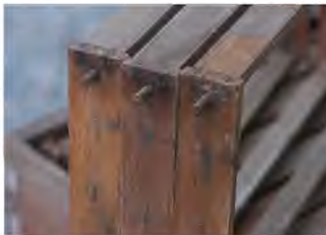
Figure 2. A closer view of the pins. Note the lack of gaps between the end bars. Consequently, these three frames could easily be handled as one piece. The end-bars also form an internal solid wall front and back.
